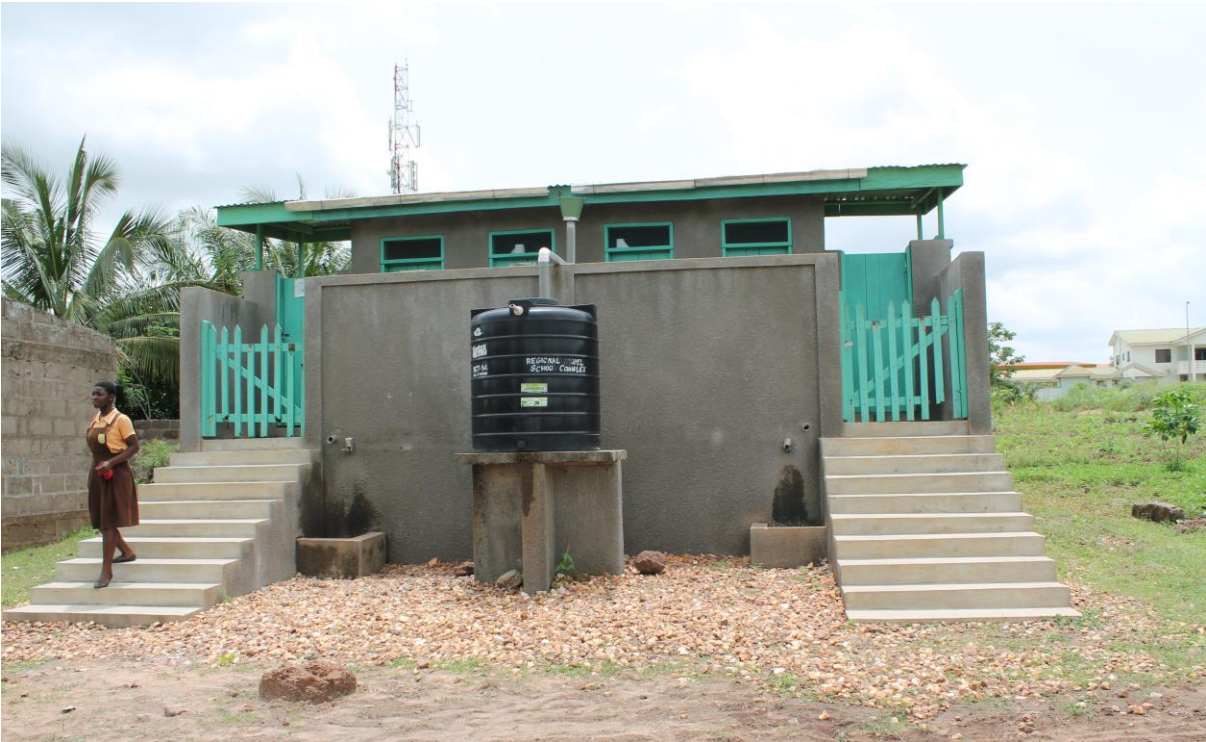
Picture 8. Urine-Diverting Dry Toilet, Ho Polytechnic Primary School
