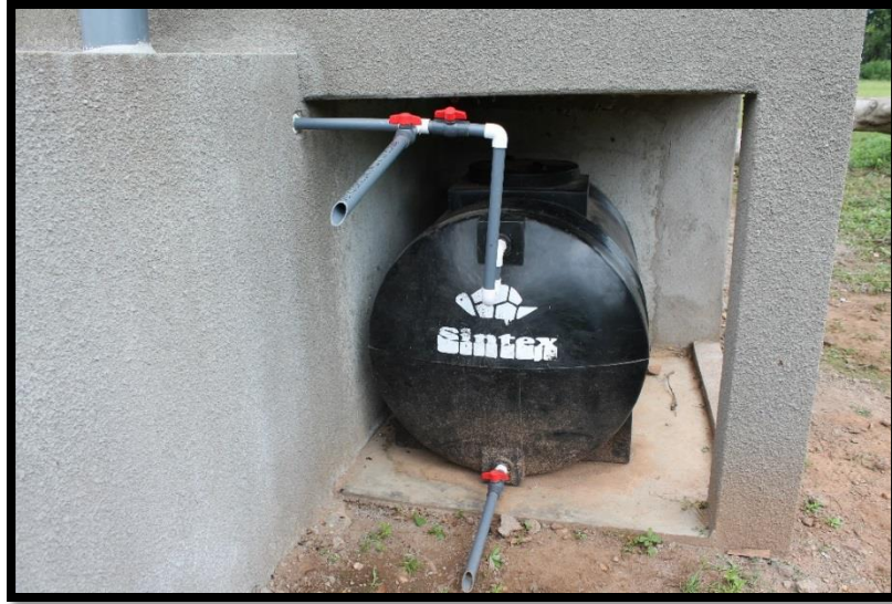
Picture 17. Urine-diversion reduces odours and enables the use of nutrient-rich and pathogen-free urine as a fertiliser (Picture: Aalto, A. 2014)
