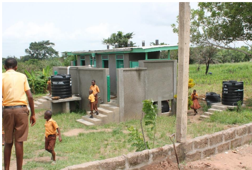
Picture 18. First urine-diverting dry toilet build at Regional Model School in 2009 (Picture: Aalto, A. 2014)
