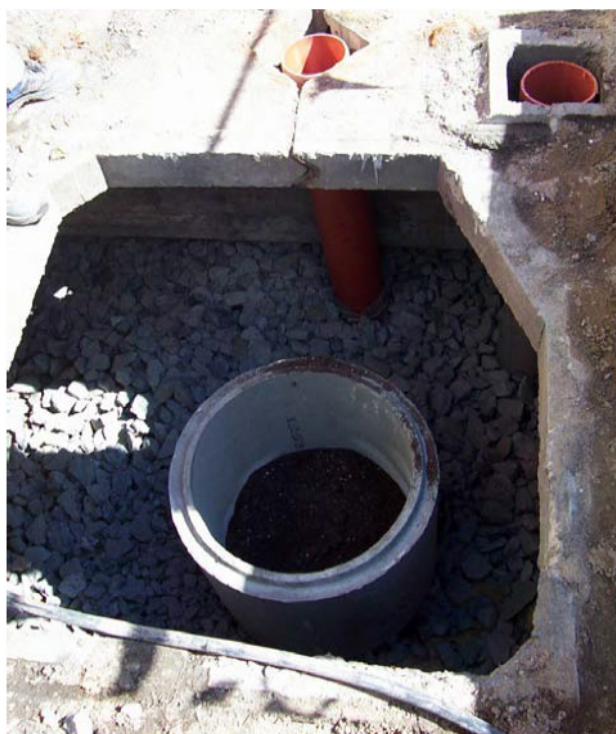
FIGURE10: Figure shows the system that is planned for street tree. (Planting beds in city of Stockholm 2009).
