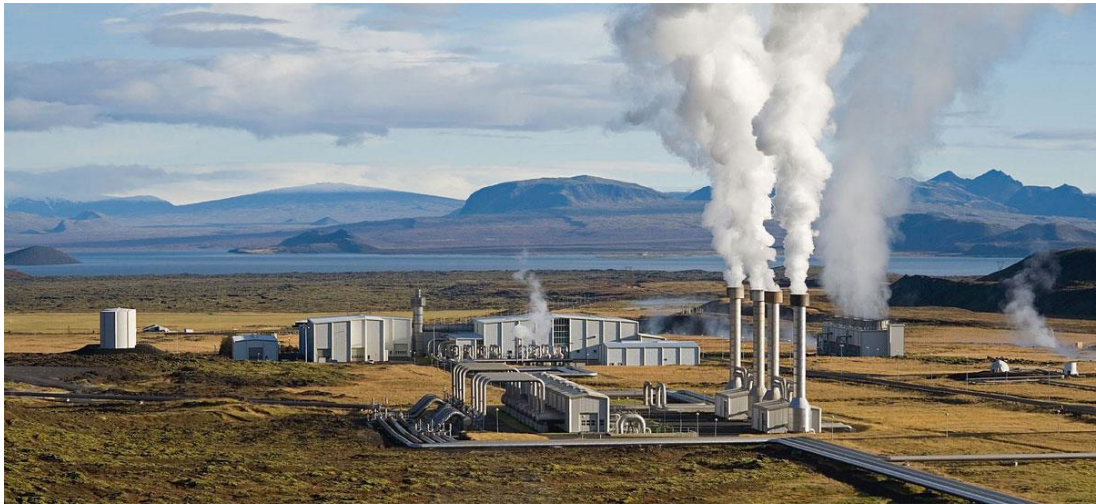
Figure 2.2. Geothermal power plant (How geothermal energy works 2014).
