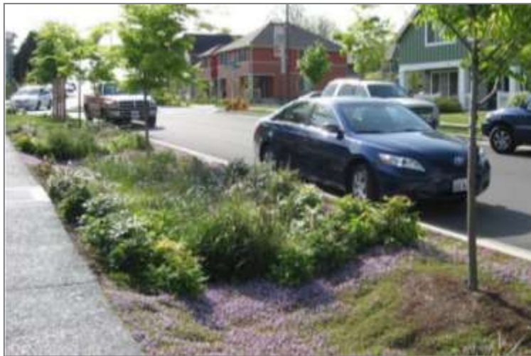
FIGURE 7. A grassed swale built between street and sidewalk (Steed 2012).
