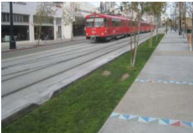
FIGURE 11. A vegetated filter strip located in the middle of a city (3 Rivers Wet Weather 2012).
