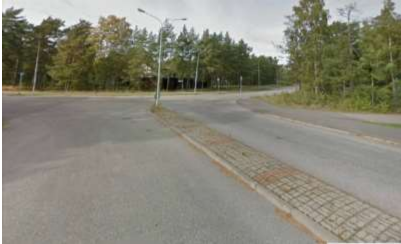
FIGURE 23. Runoff water has nowhere to be absorbed (Google Maps 2014).
