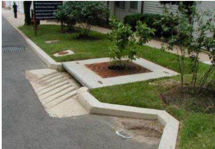
FIGURE 9. A newly built tree box filter (Steed 2012).
