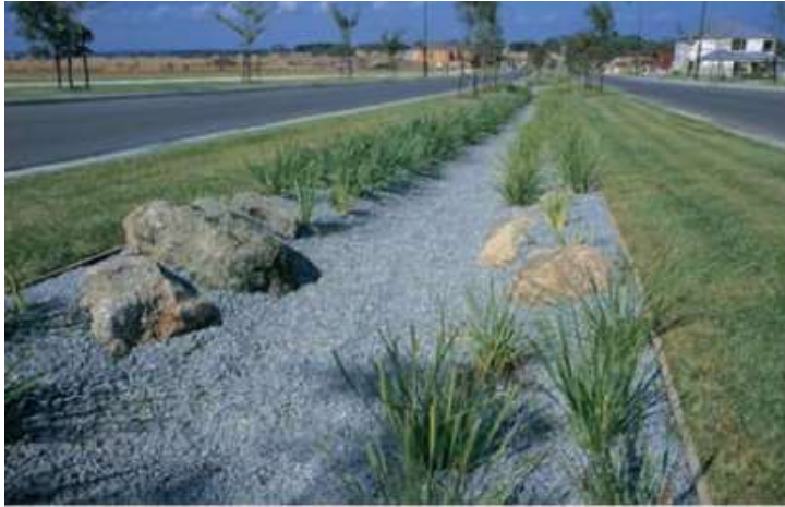
FIGURE 10. An infiltration trench located in the median strip (Steed 2012).
