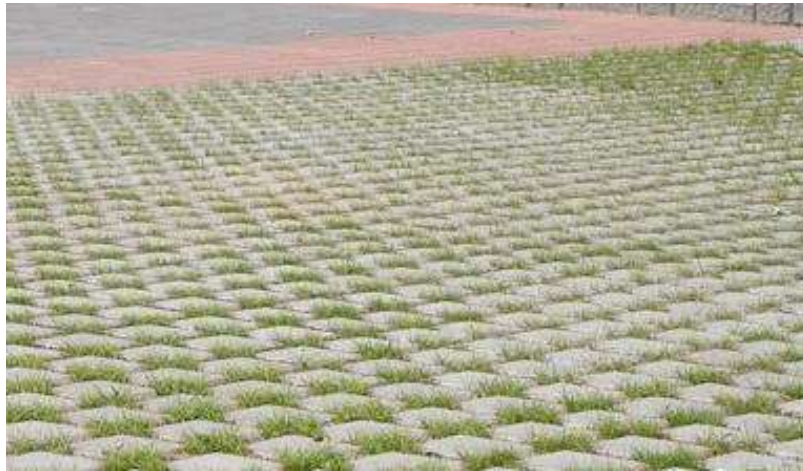
FIGURE 8. The structure and form of pervious pavement is planned to direct rainwater through the grass growing in between of the paving (HB-Betoniteollisuus Oy 2013).
