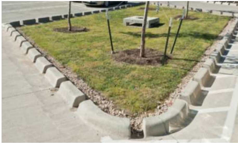
FIGURE 4. The amount of curb cuts can be adjusted according to the need. Here is an example from Seattle (Feliciano 2015).
