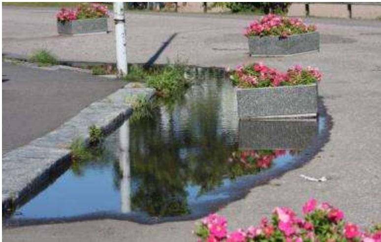
FIGURE 26. An example of how water cannot penetrate impervious surfaces but flows downhill to the lowest point (Komulainen 2014).
