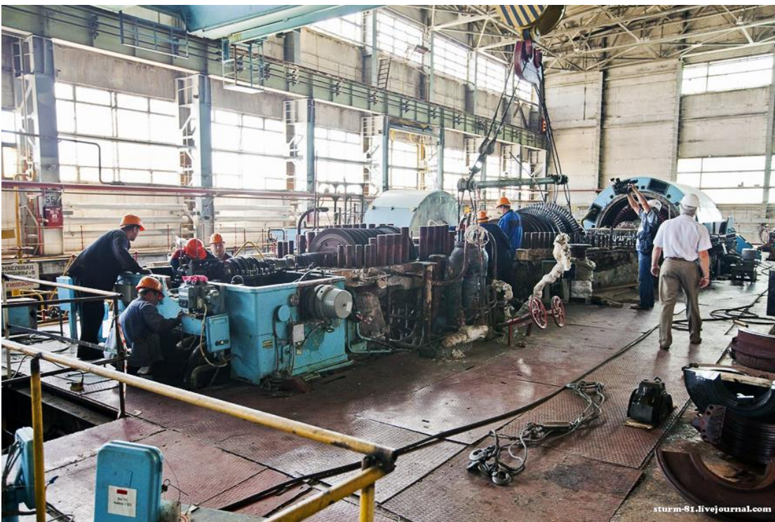
FIGURE 14. Capital repairing of turbine CHP-2 Ufa. (CHP Ufa, 2012)
