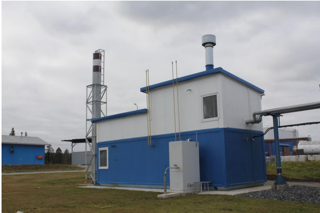
Figure 3. ZAO “Sibirit -3”; boiler house, Kostomuksha, Russia. (Vladimirov Vladimir)
