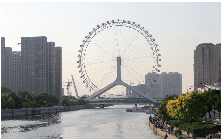
Tianjin Eye, a 120-metre tall giant observation wheel built above the Yongle Bridge, over the Hai River in Tianjin. Photo: Anu Härkönen
