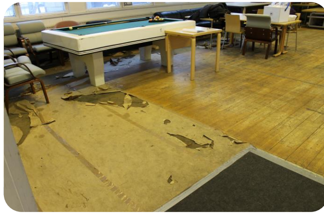
FIGURE 15. Second sampling area of building P
