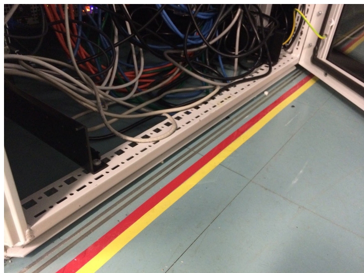
Figure 8: Water leak sensor
