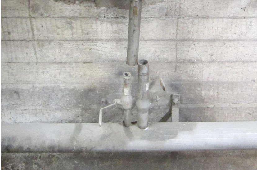
Picture 25. Cut pipes under curing area in cellar floor
