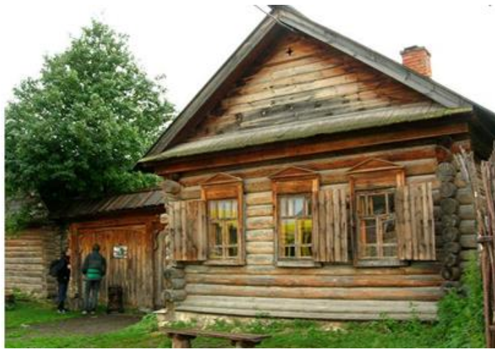
FIGURE 2. Typical houses for Shiryaevo village.
