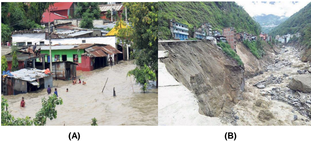
Figure 5. Types of riverine floods: (A) Gaidakot in Nepal after the Narayani river overbank flooding in 2016 (7) and (B) Buildings and Roads in Nepal Swept by the Bhotekoshi river flash floods in 2016 (8)
