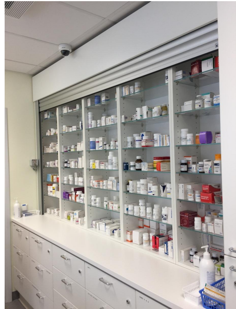
Medicine cabinet Surgical Rehabilitation Ward T6
