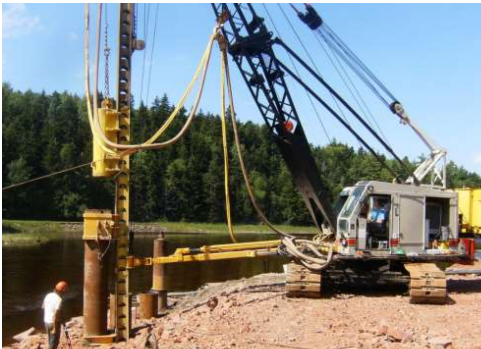
Figure 13. Drop hammer. (Heavy Civil Construction, 2016)
