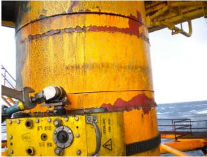
Figure 28. Water jet cutting above water level. (External Abrasive Waterjet Cutting, 2016)
