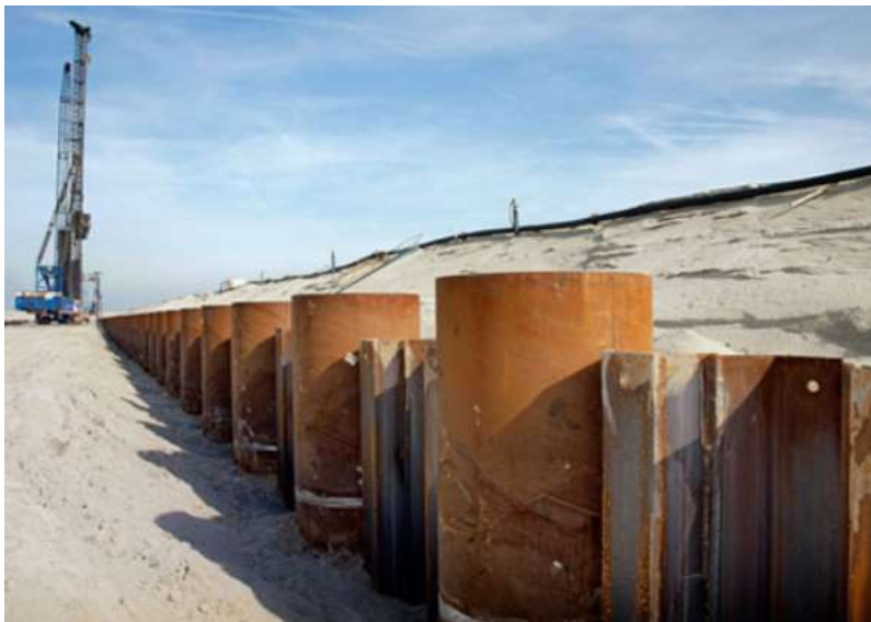
Figure 11. Combi-wall. (SSAB, 2017)
