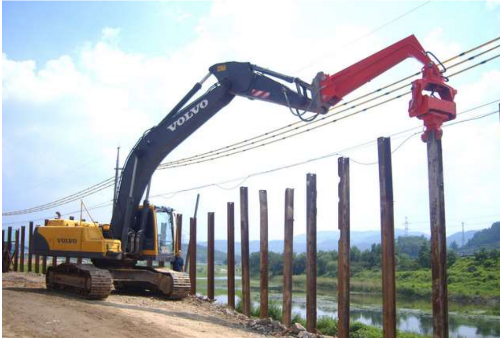
Figure 17. Vibratory hammer. (DAEDONG Engineering, 1996)
