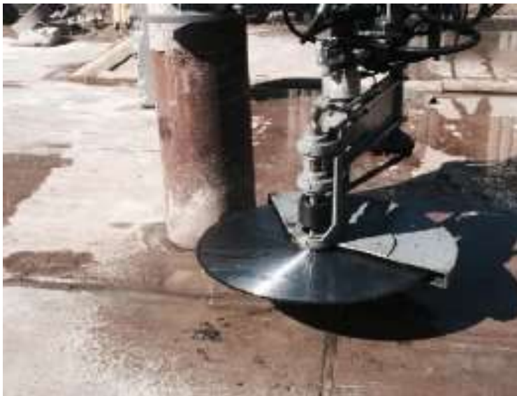
Figure 26. Pile Cutting Machine of Aggregate Technologies (Cutting Steel Piles)
