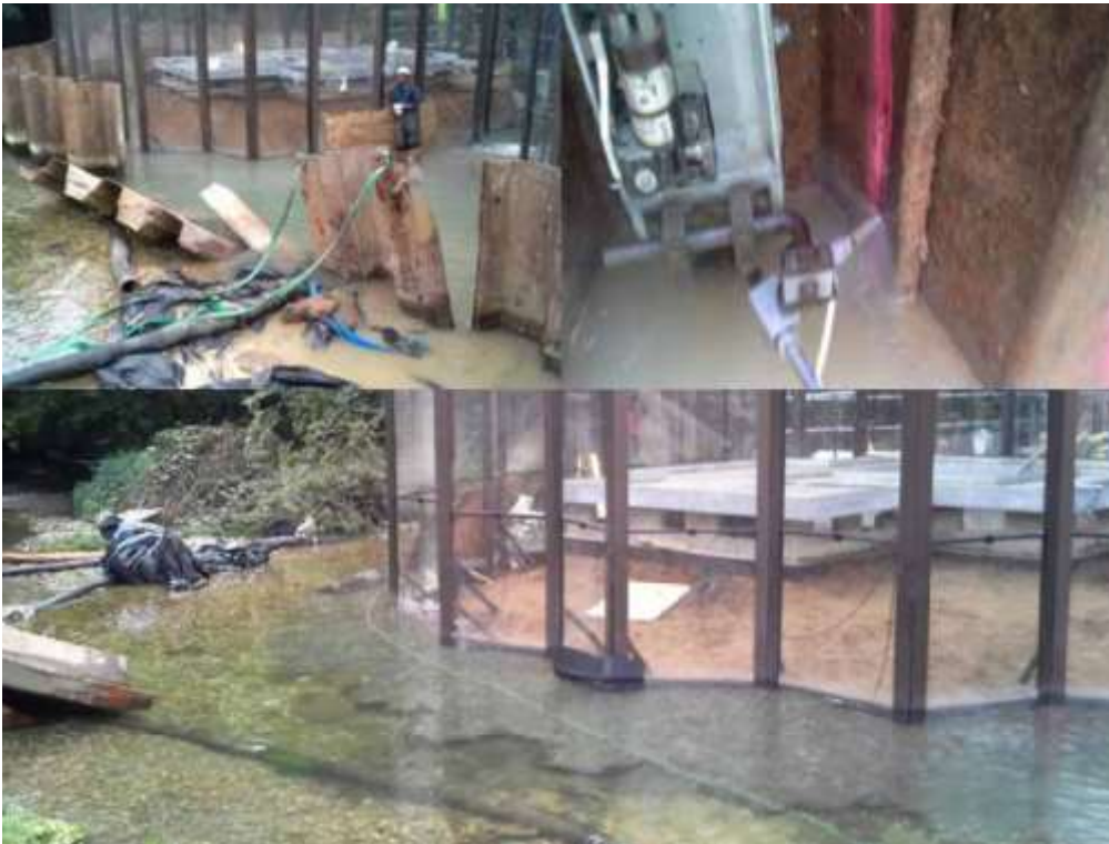
Figure 39. Phases of cutting and the final outcome. (RGL, 1998-2013)
