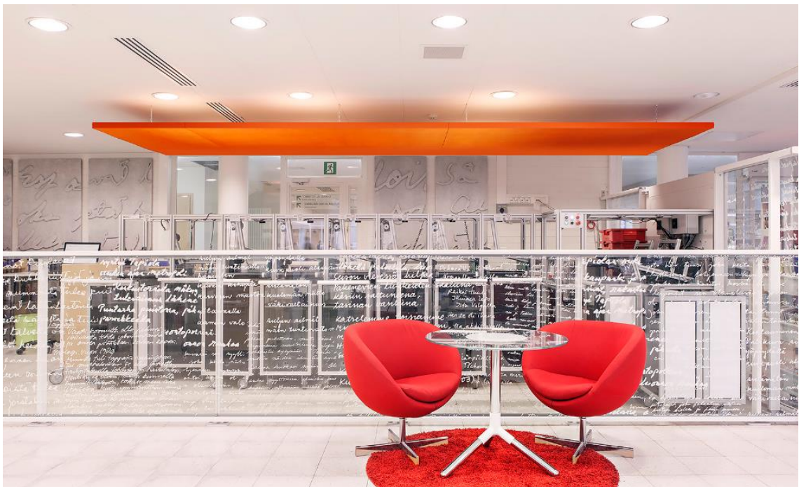
Figure 12. Functional and colourful ceiling panel installation off the ceiling (Hyppölä, 2016).
