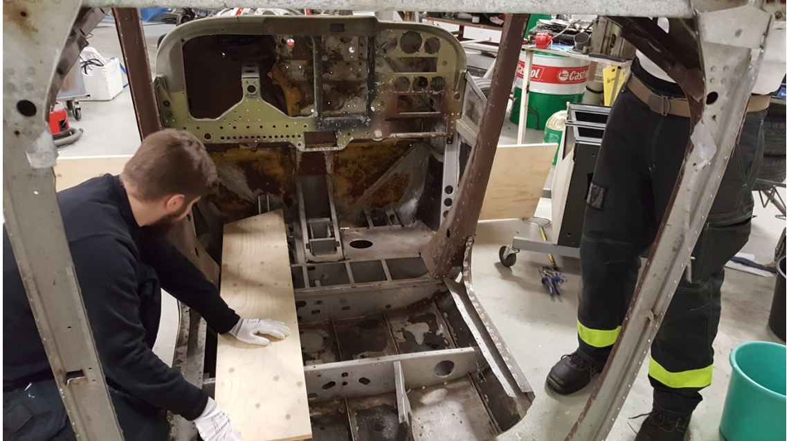
Picture B.3 Project members working on the adjustment of the cockpit. The inner modifications include the installation of cockpit instruments in the front panel as well as the structure enhancement. In the picture project members are working on the adaptation of the cockpit floor. (Photo: Jarno Puska 2016).
