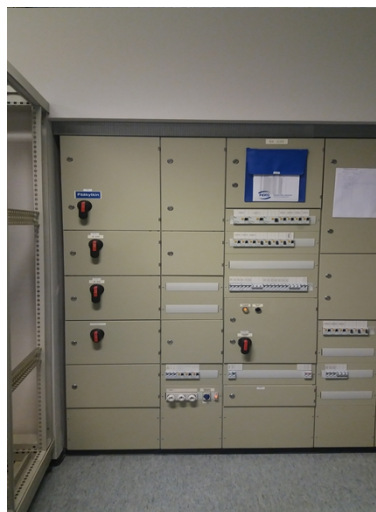
Picture 3.3 Panel of emergency buttons in one of TAMK's laboratories. (Photo: Berta Martínez 2017).
