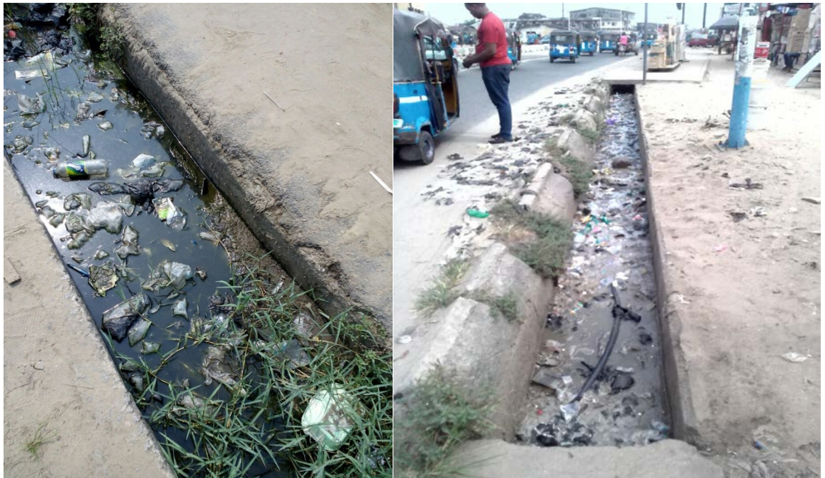
Figure 2: Pure Water bags amongst plastic containers blocking drainages in Osubi Town (Ekrake, 2015)
