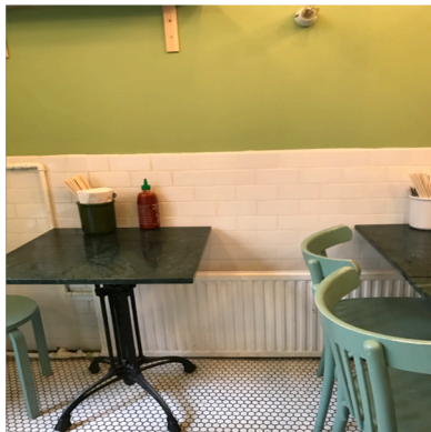
Figure 9 Vibami - heating system
