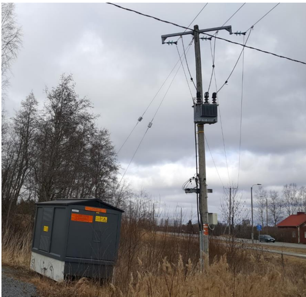
Figur 6, KL-INDUSTRI SatElit marktransformator
