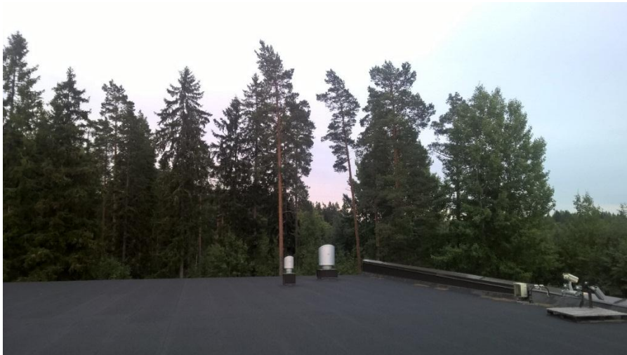
Figure 6 Picture from the roof towards the south (Author, 2016)
