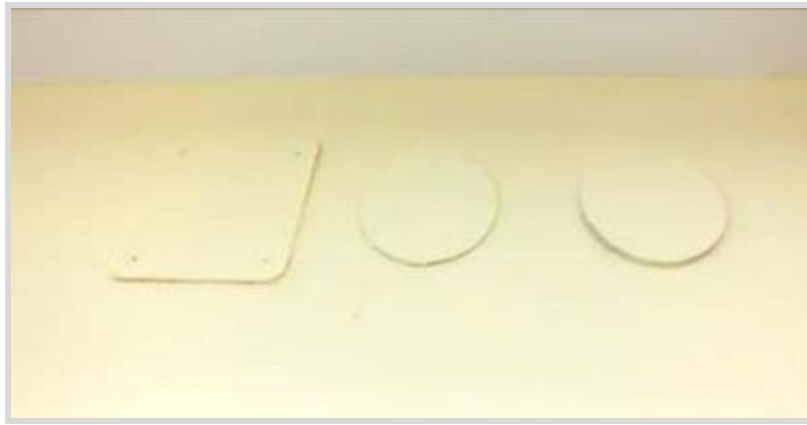
Figure 5: Hatches are subtly colored not to be intrusive to the overall design (Poznan University of Economics)
