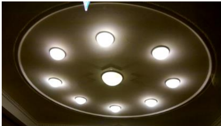
Figure 23: Ceiling light fixtures installed in accordance with the decorative carvings (seen in University of Tuebingen)
