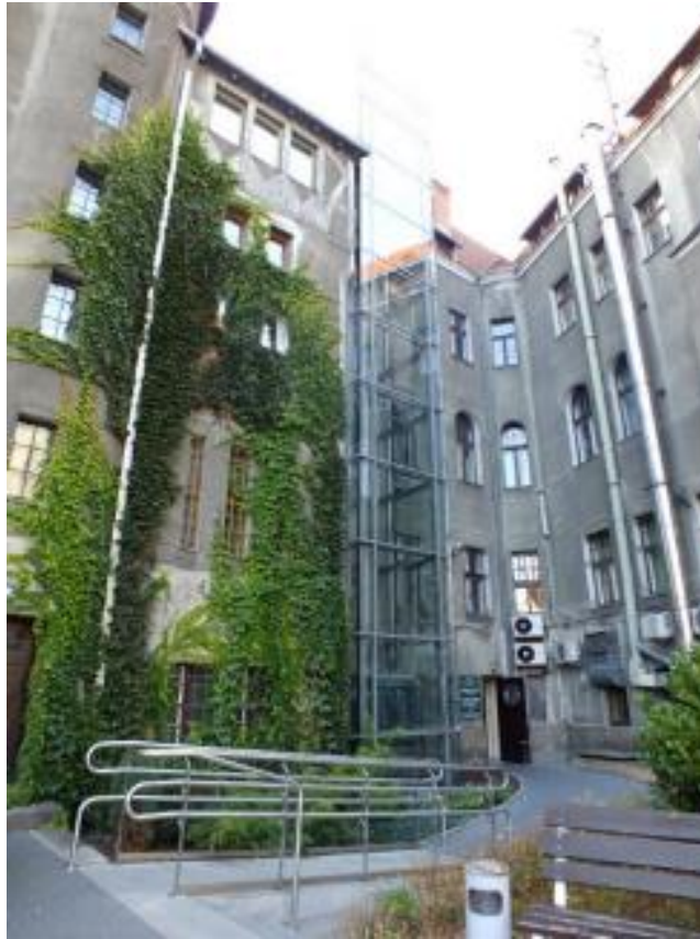
Figure 20: The elevator of Poznan University of Economics from the outside
