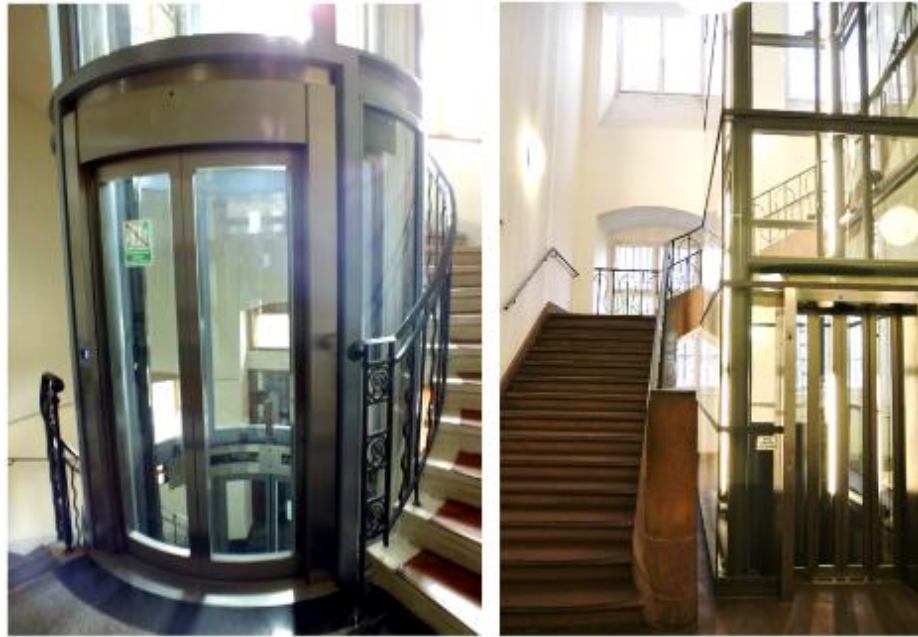
Figure 18: Elevator installed in the available space of an original spiralling staircase, partially removed to create entrance (left: Adam Mickiewicz University, right: University of Mannheim.)
