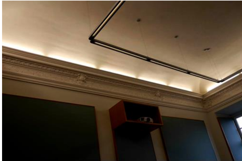
Figure 26: The combination of ceiling fluorescent lights and hidden bulbs in the decorative panel, as seen in University of Mannheim.
