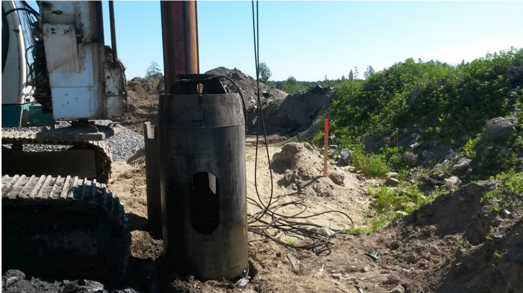
Image 1. Drilling of sampling hole in Metsäsairila landfill in June 2016 (photo by Ramboll Finland Oy)
