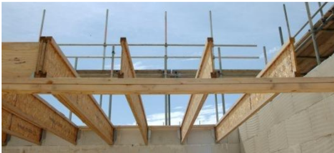
Figure 3.9 Example of flooring system with Finnjoists. (Finnforest).
