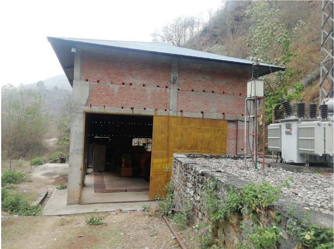
Figure 4. Transmission of electricity from the powerhouse.
