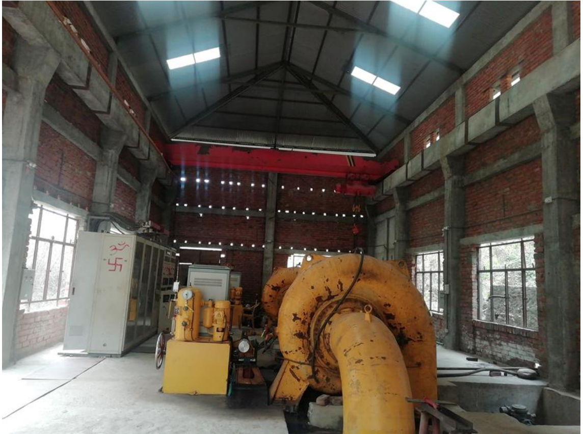
Figure 3. Walls, roof and lighting inside the powerhouse.
