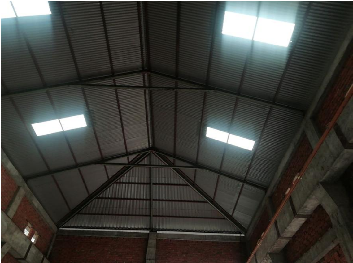
Figure 1. Roof of the powerhouse.
