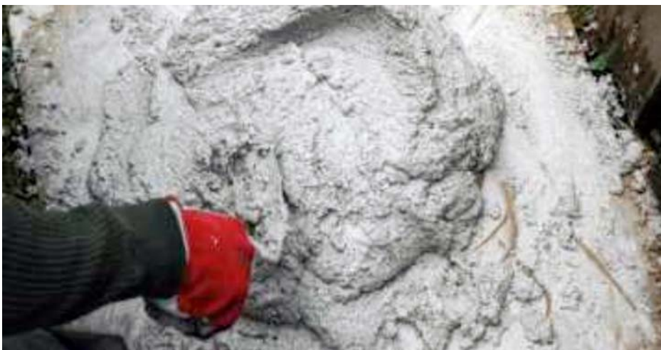
Figure 10. Mixing hot lime by hand.
