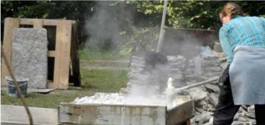
Figure 11. Wet slaking. Kristin Balksten in action.
