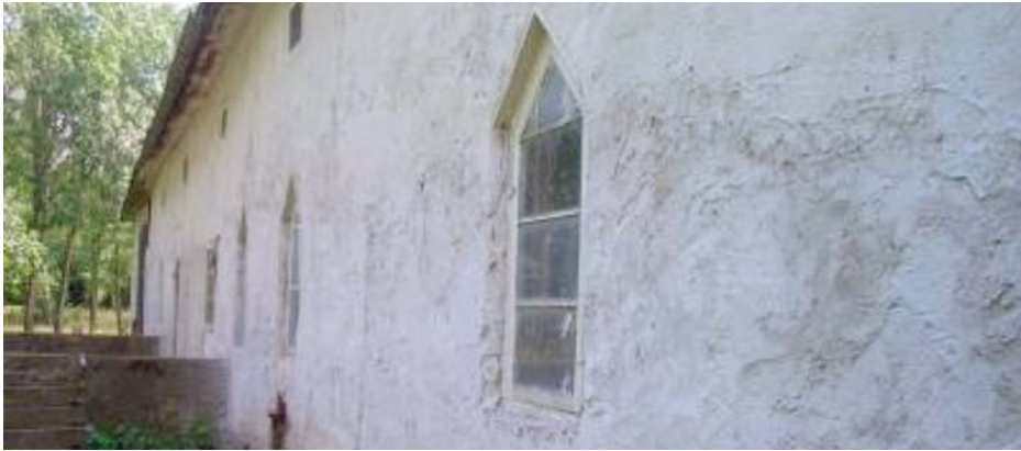
Figure 16. The facade with patches of student work.
