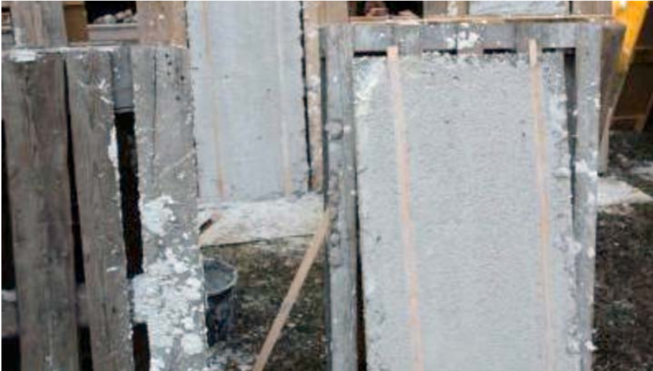
Figure 14. Creating an even surface by using two strips of wood as guide.
