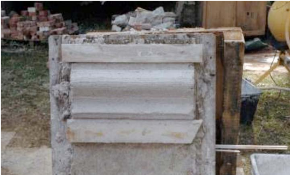
Figure 15. Moulding the surface by using a stencil.
