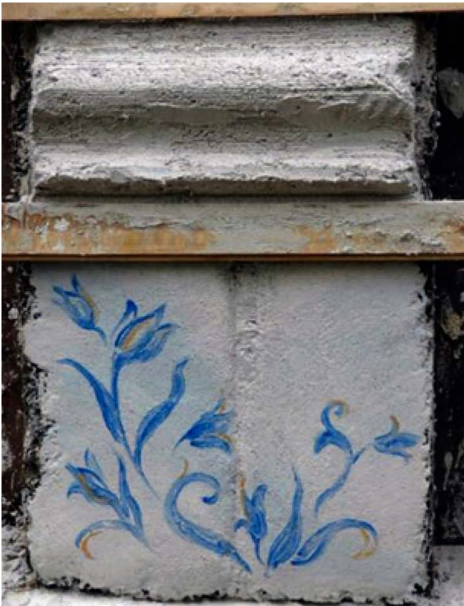
Figure 5. Lime wash can also be used for decorative purposes. This little experiment was made by one of the students in al secco technique on dry plaster.
