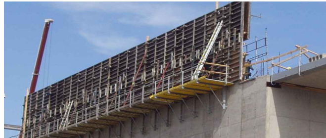
Figure 13 Large unit of sheeting panel form system
