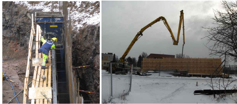
Figure 19 Concrete bucket and concrete pump used to pour a wall structures
