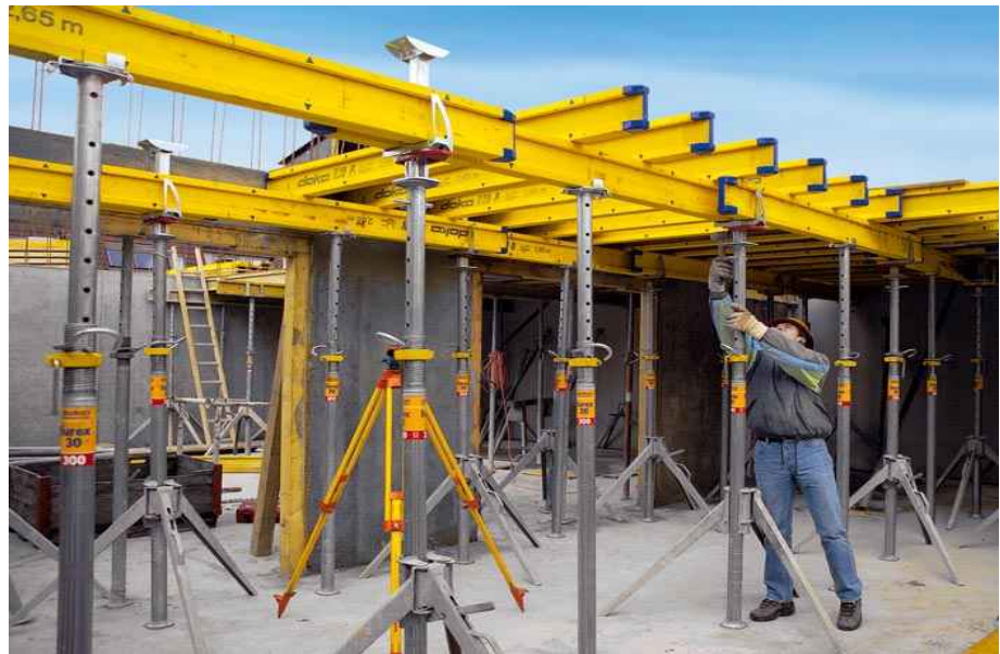
Figure 17 Installation of standard beam form system
