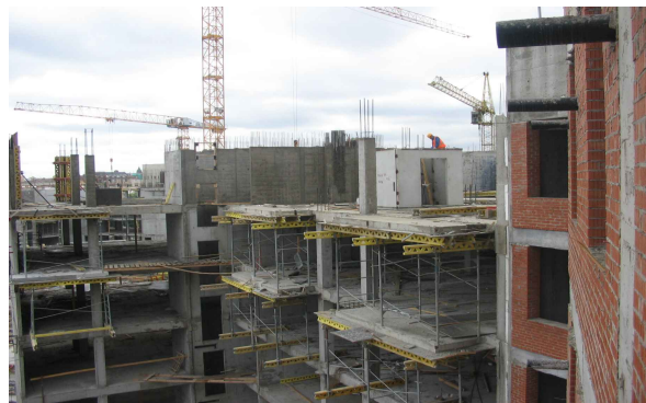
Figure 7 Column slab frame under construction in St. Petersburg
