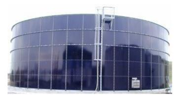
Figure4. Biogas reactor made of steel with fused glass coating[11]
