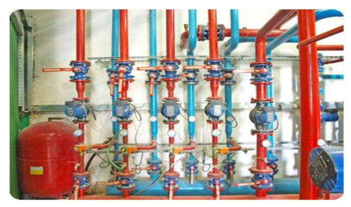
Figure 10. Heating unit of biogas plant [16]
