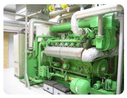
Figure15. Biogas co-generation heat power unit [21]
