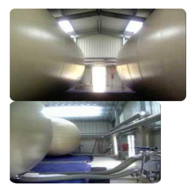
Figure 9. Gas holder in special hangar [15]
