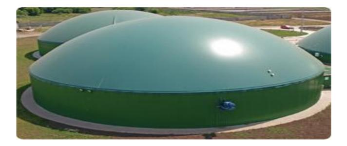
Figure8. Gas older for biogas [15]
