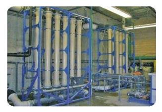
Figure 21. Membrane module in operation [23]
