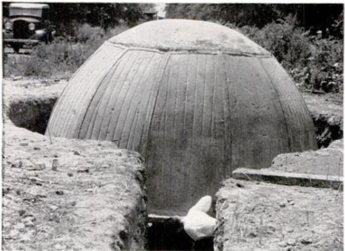
Concrete pillbox , made of quick-drying concrete, was constructed for Army demonstration by its inventor, Karl Billner of Philadelphia, took only five hours to build.
