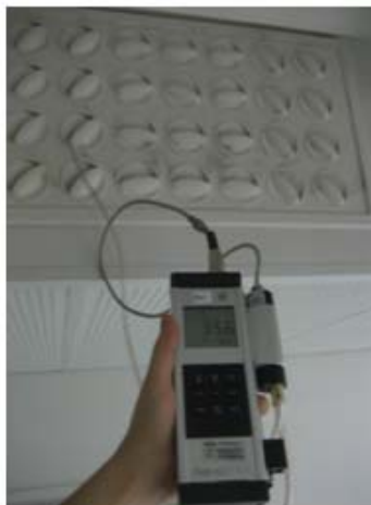
FIGURE 13. Measuring pressure in supply air distribution device by Swema Air 300
