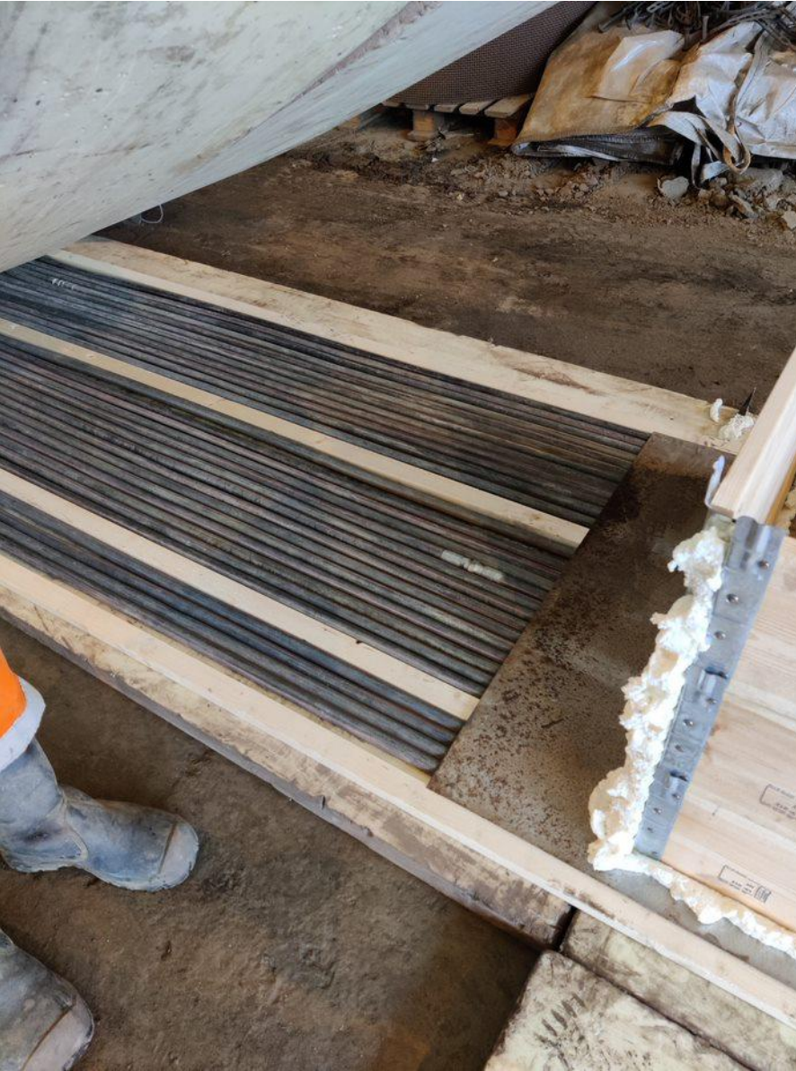
PICTURE 3. Hot oil tubes under the aluminium plates.
