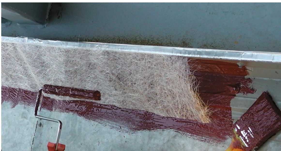
Figure 3. Application of Sika MTC system
