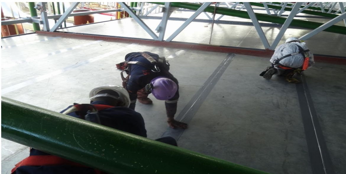
Figure 12. Application of bridging tape over roof element joints.
