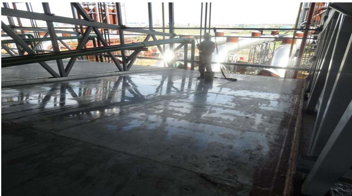
Figure 11. Solvent cleaning of roof elements
