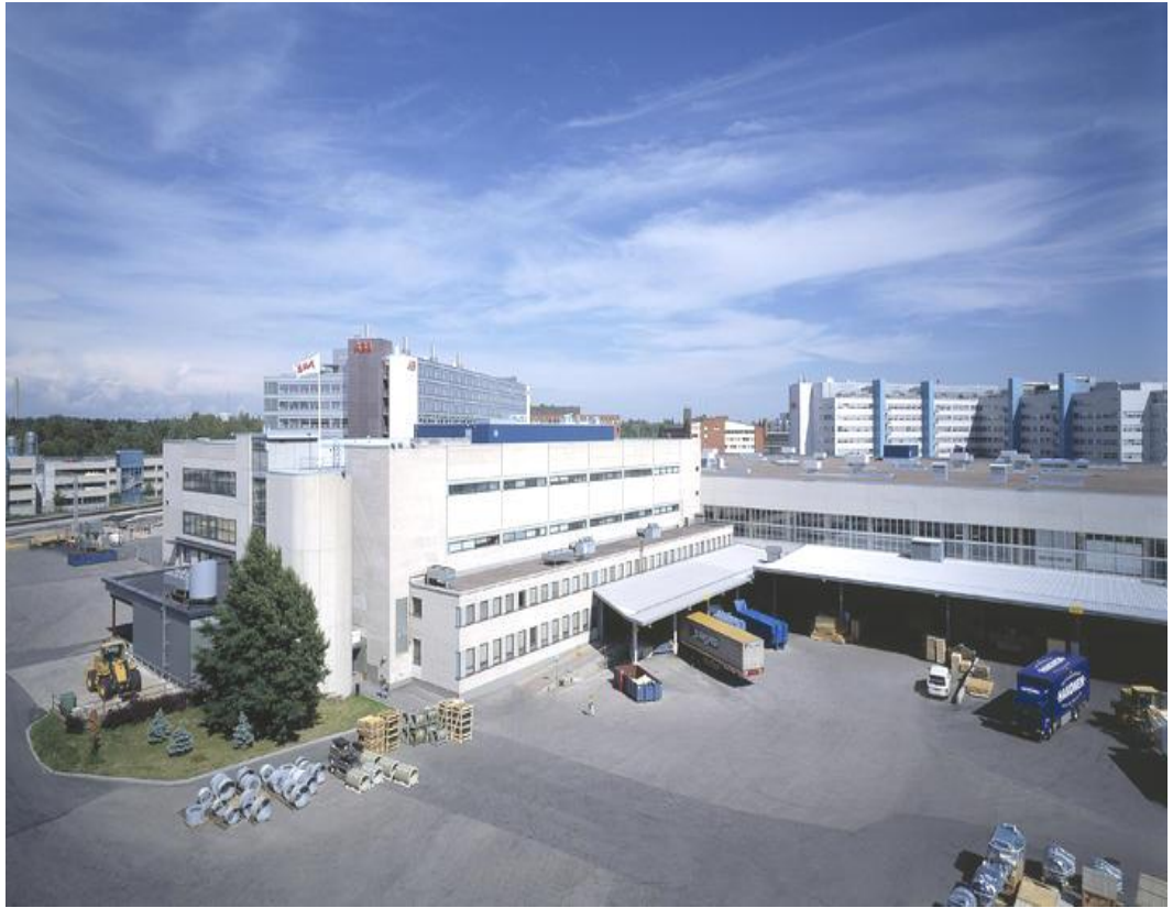
FIGURE 3 ABB Drives & Controls, Helsinki. (ABB,2013)
