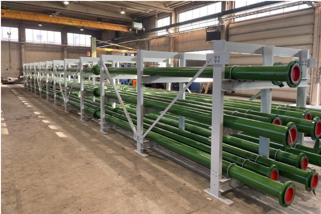
Figure 5. Installation and alignment at the workshop. (Wärtsilä 2022.)
