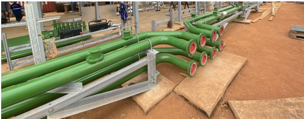
Figure 1. Prefabricated cooling water pipes. (Wärtsilä 2022.)
