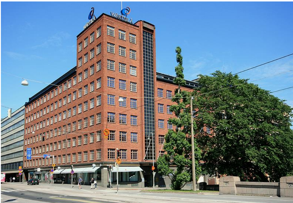
Figure 1. Wärtsilä headquarters in Helsinki. [2]
