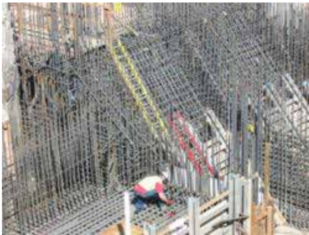
FIG 34 Rebar for foundations /22/
