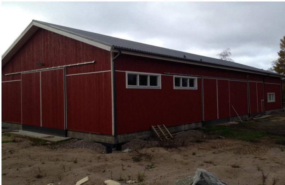
Figure 1 Outside view of the building
