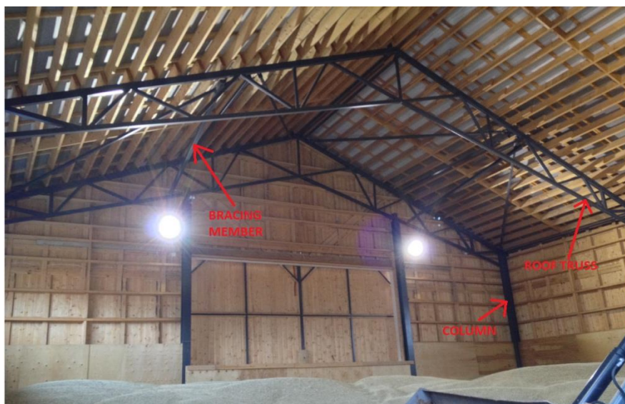
Figure 2 Interior truss members
