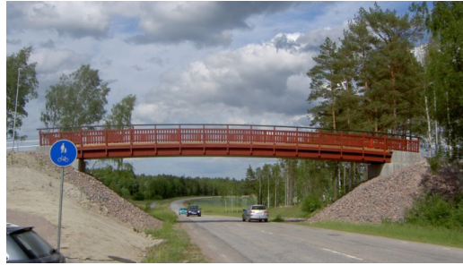
Figure 5 pedestrian bridge, box-beam bridge with a span of 24,5 m, Nyköping, Built in 2007. Photo: Moelven Töreboda AB.
