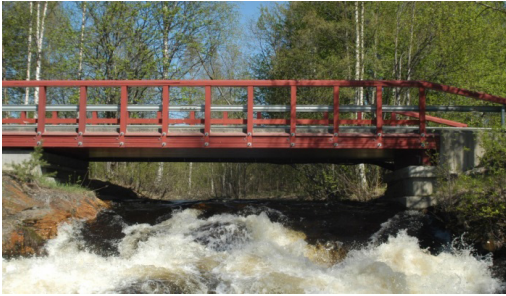
Figure 4 Stress laminated timber road bridge, Klintforsån, Skellefteå, built in 1999. Photo: Per-Anders Fjellström
