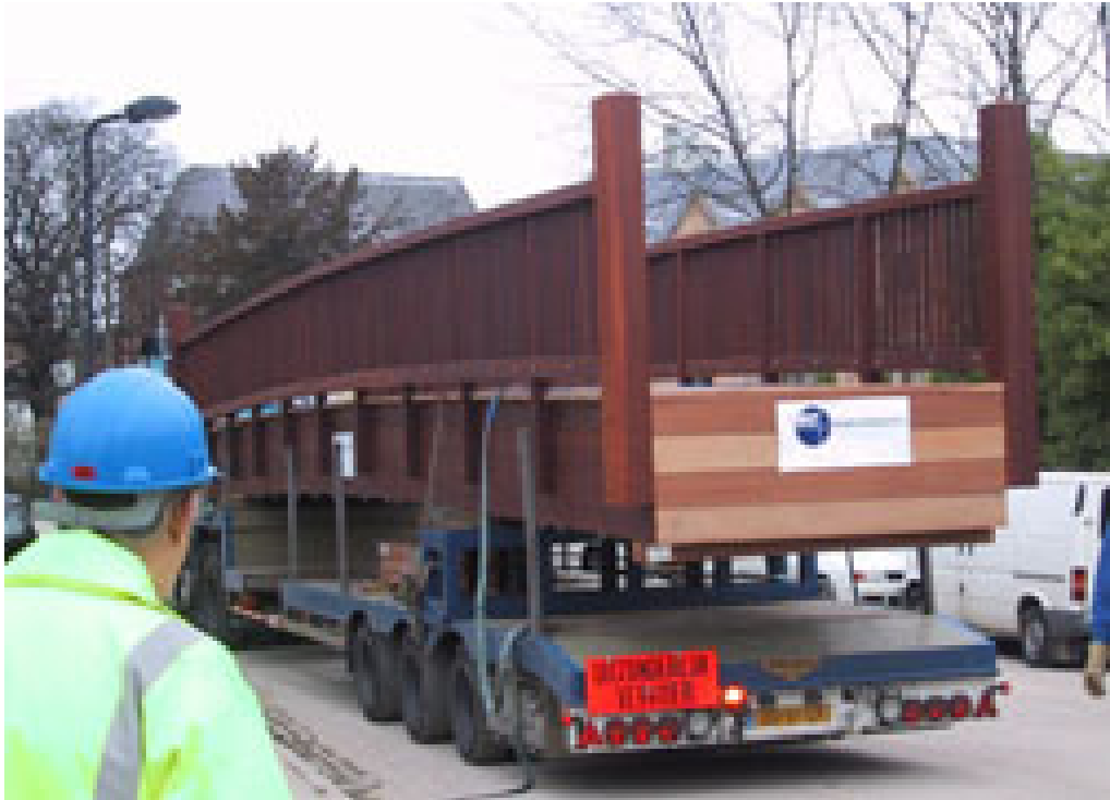
Figure 16 Erection of a pedestrian bridge, Photo Martins Child Limited
