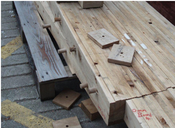
Figure 15 SLT-bridge solution. Photo: Anders Gustafsson
