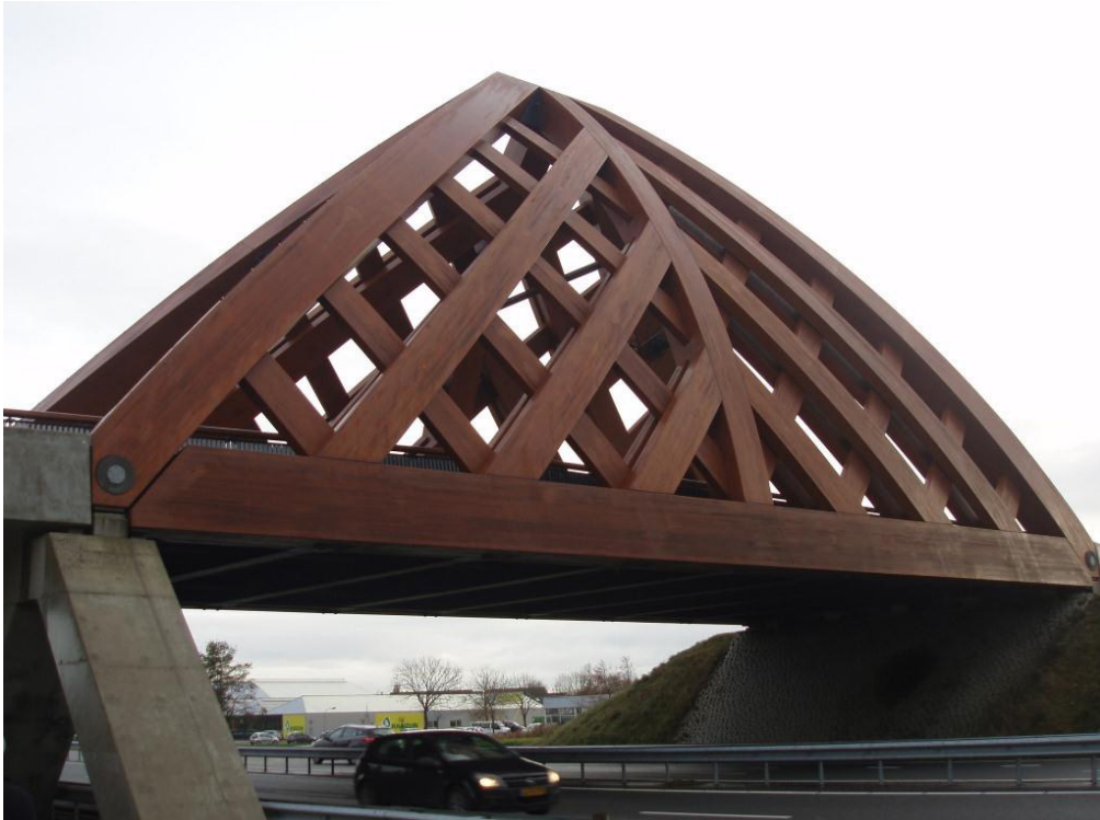
Figure 14 Bro Sneek, full traffic load bridge. Photo: Anders Gustafsson
