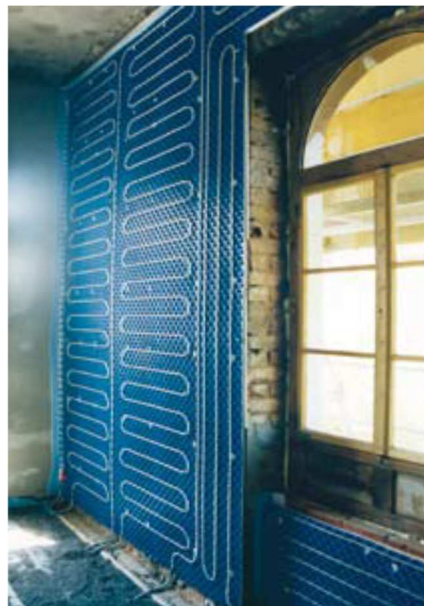
FIGURE 8. Example of heating panels installation to the walls /11/
