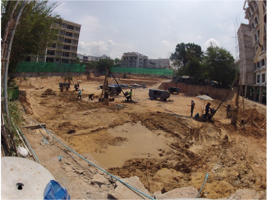
IMAGE 4. Piling work from the Tropical Garden project (Kuronen and Turunen 2014-07-24).
