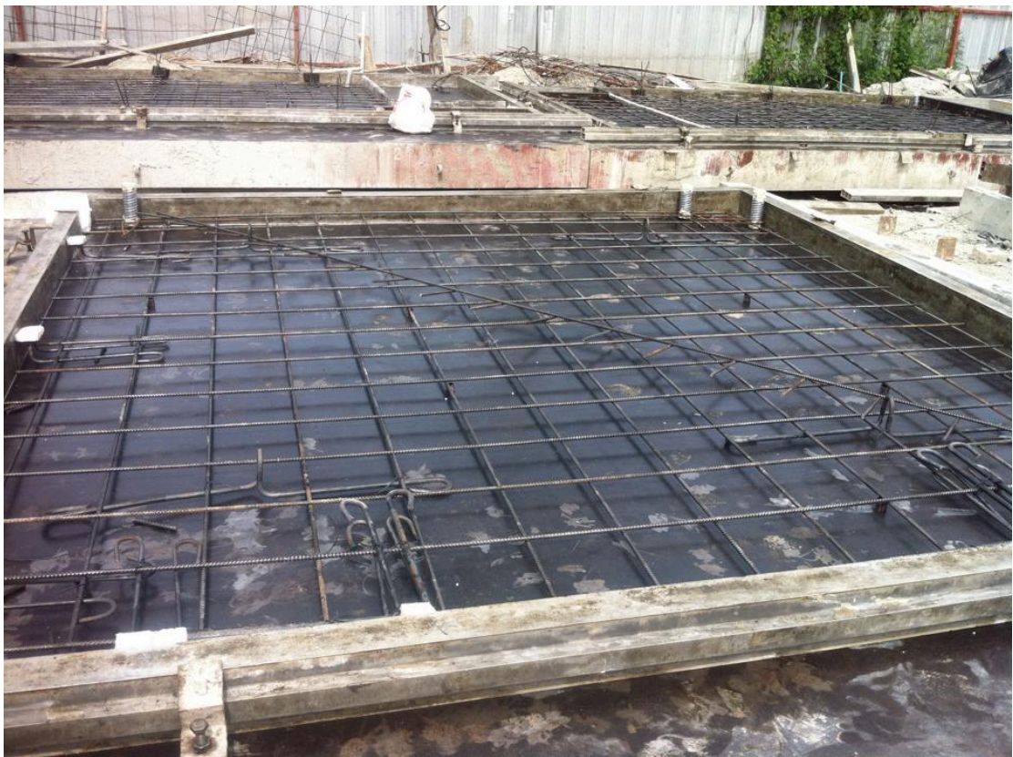
IMAGE 12. The reinforcements of loadbearing wall in the Pro-Buid factory
