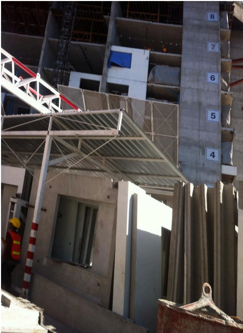
IMAGE 10. Exterior walls precasted on Pre-Built Public Company Limited's construction site
