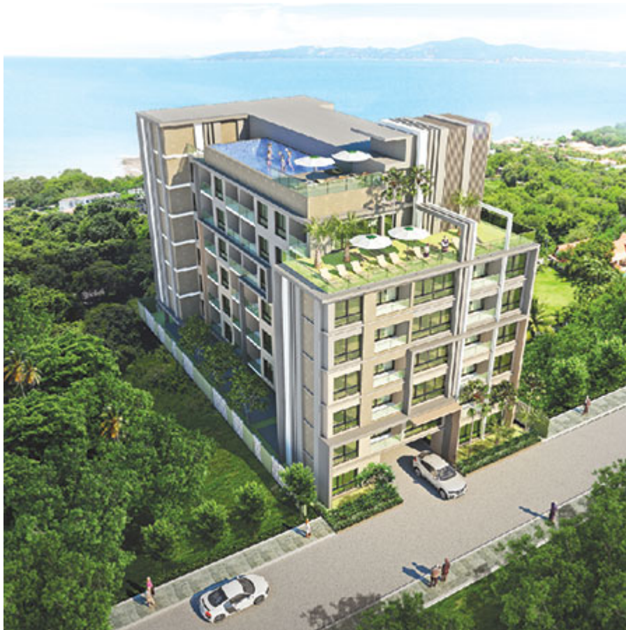
IMAGE 15. One of the completed projects of Scanditech (siamoriental.net)
