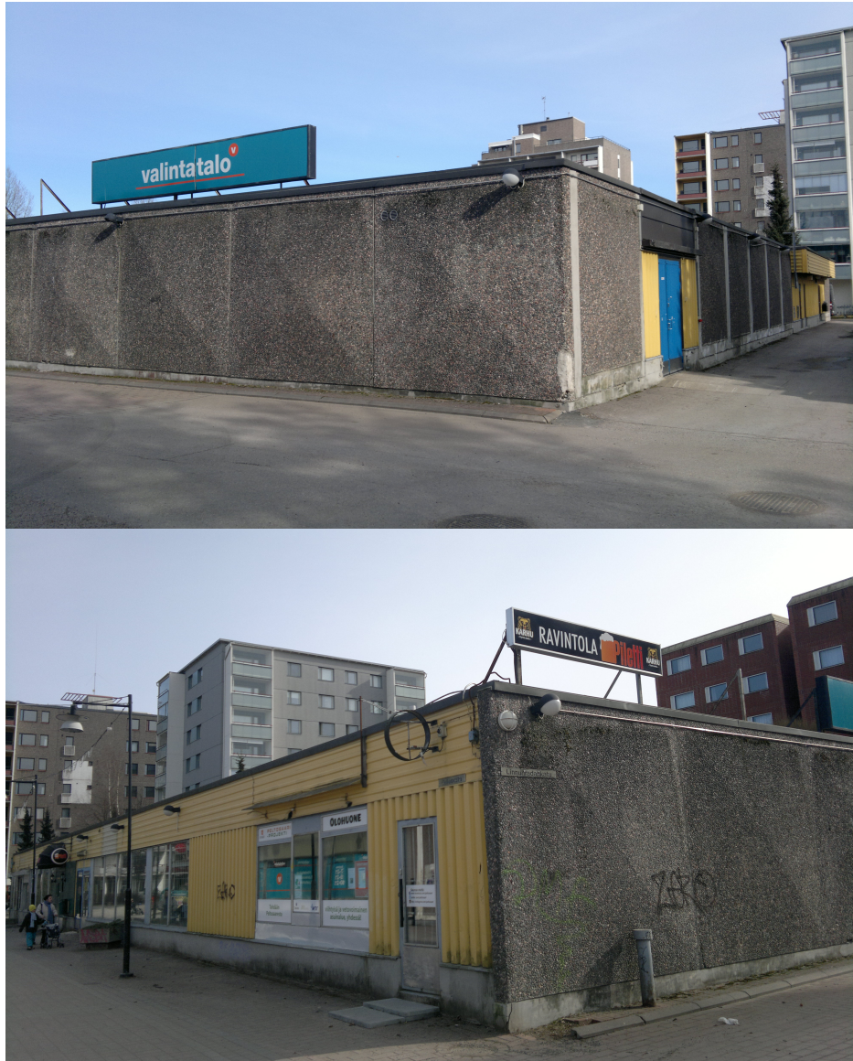
Figure 3 Outside appearance of the building
