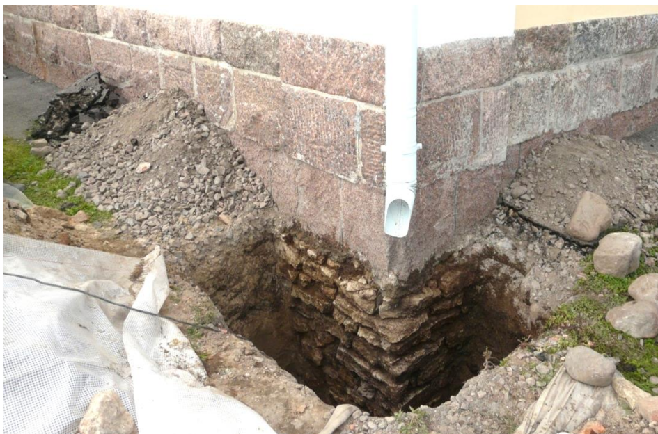
Figure 10.19 Peterhof. The Museum of the Imperial yacht. Foundation masonry made of limestone. Socle made of granite blocks to the lime-sand mortar or embedment of the masonry seams by plumbum. Blind area made of asphalt
