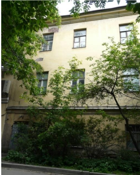
Figure 10.24 Saint-Petersburg, Sadovaya Street, the house 8/7
