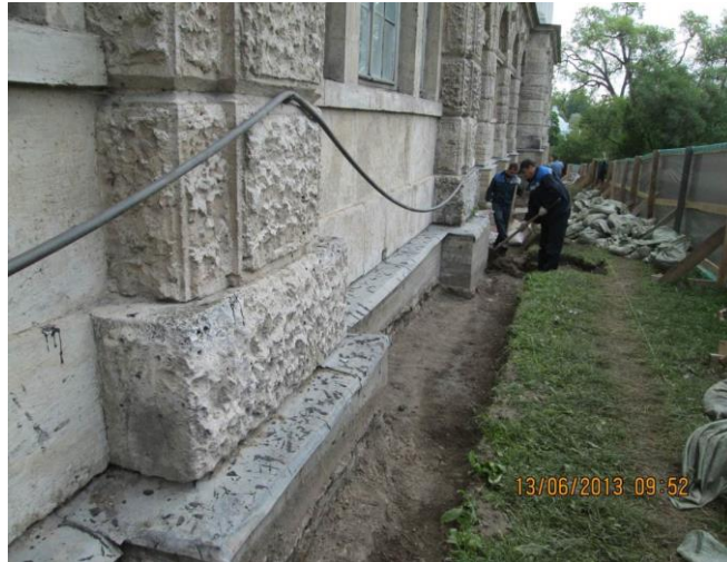
Figure 11.6 Phased digging of soil along the building
