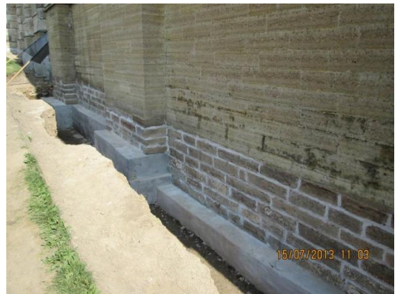
Figure 11.8 Application of waterproofing covering
