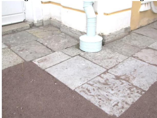
Figure 10.17 Peterhof. Grand Palace. Socle made of sawn limestone to the lime-sand mortar. Blind-area made of limestone. Heated outfall from the roof into the sewer network
