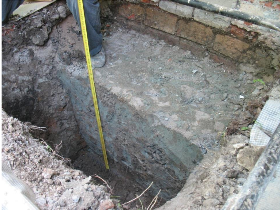
Figure 10.3. Kamennoostrovsnyi Palace. Foundation waterproofing by the clay lock
