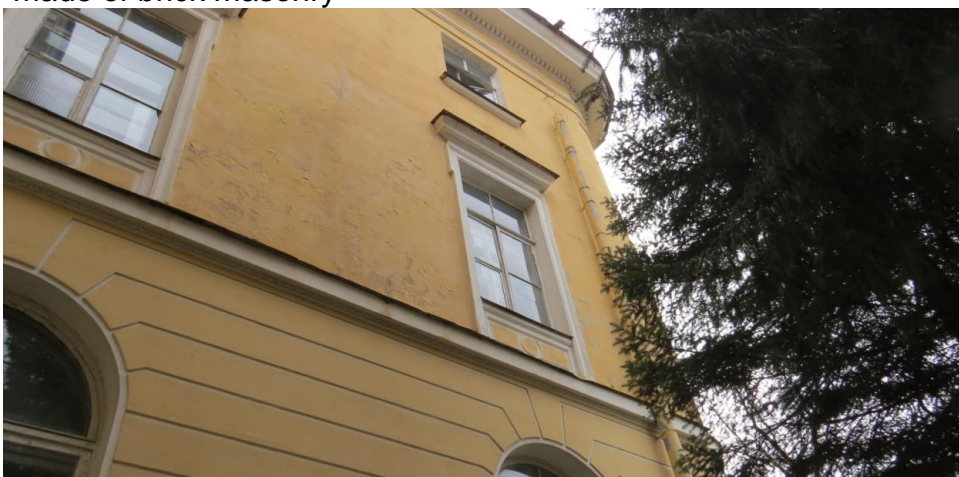
Figure 10.34 Pushkin. Paley B.G. Palace. Main and secondary cornices made of brick masonry, cornices above and under the windows made of steel sheets
