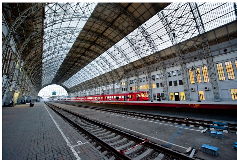
Figure 2.6 Frame-arch structure of Kievskii railway station in Moscow. (Wikipedia website)
