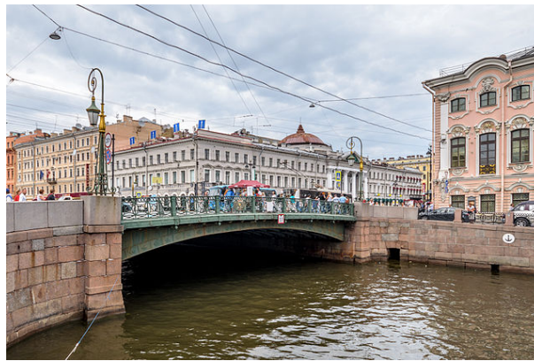
Figure 2.3 The first cast iron bridge in Saint Petersburg. (Wikipedia website)
