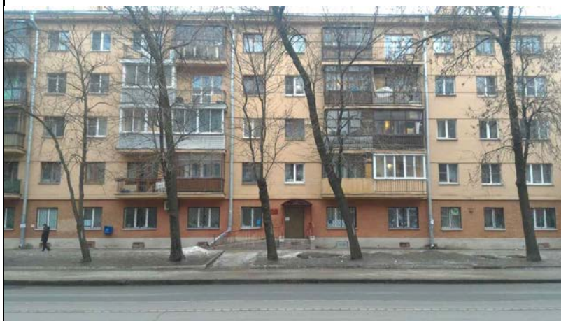
9 Facade with reconstructed entrance group
