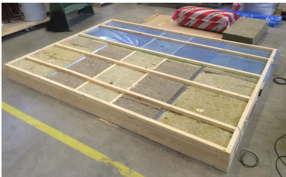
Figure 10. Wall construction in process
