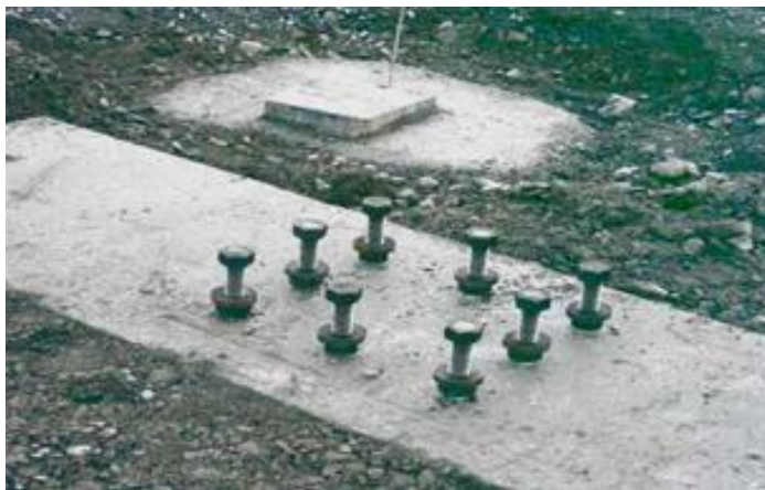
Figure: 50 Installed anchor bolt (2017, FK Bud llc)
