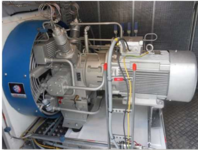
Image 6 - NG1 compressor installation
