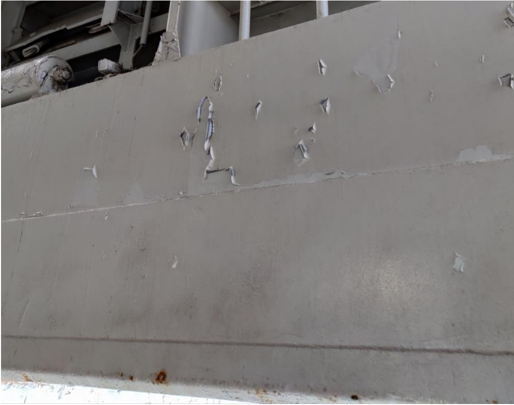
Figure 26 Loose paint on hatch cover. (Matti Heinonen 2021)
