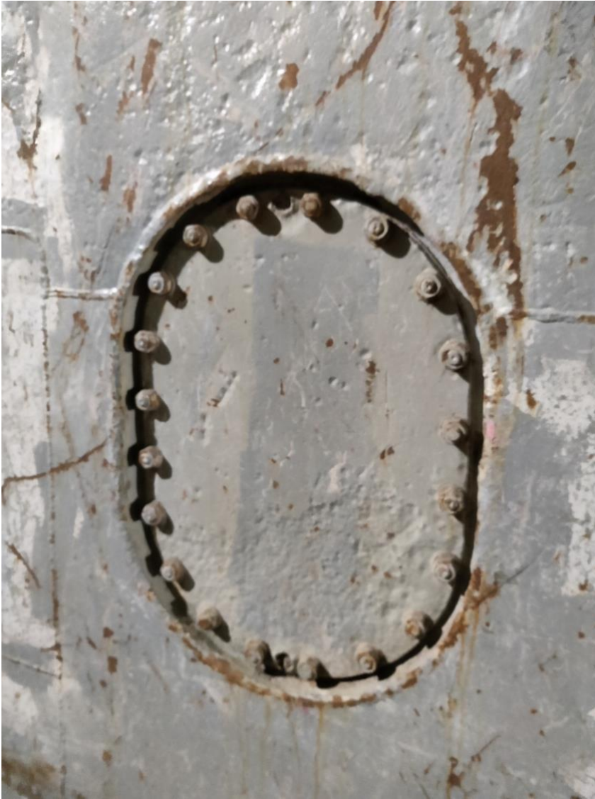
Figure 16 Side plating manhole (Matti Heinonen 2021)
