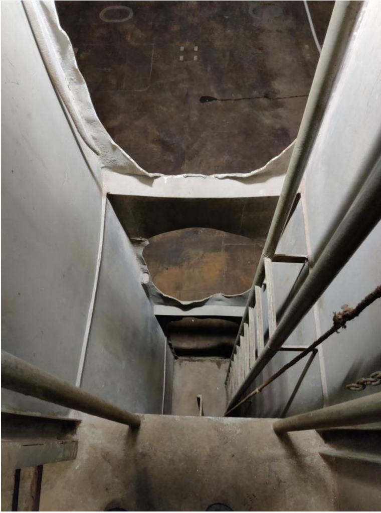
Figure 23 Aft cargo hold ladders and housing. (Matti Heinonen 2021)
