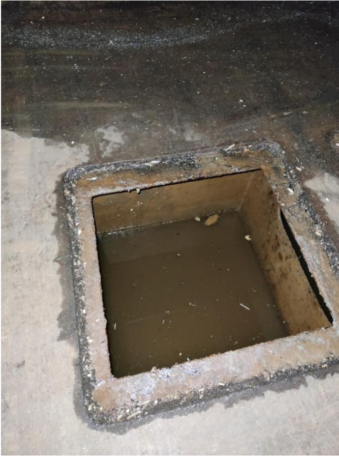
Figure 15 Bilge full of water after washing that needs to be cleaned (Matti Heinonen 2021)
