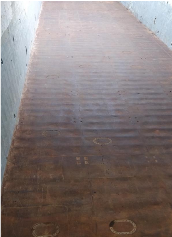
Figure 14 Clean and dry tanktop (Matti Heinonen 2021)
