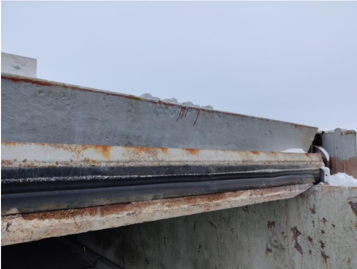
Figure 30 Hatch cover sealing gasket from mid-ship. Sealing between aft and forward hatch covers. (Matti Heinonen 2021)
