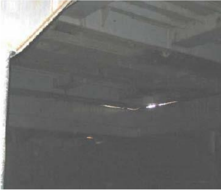
Figure 10 Light infiltration test (Bulk Carrier Guide, 2010)
