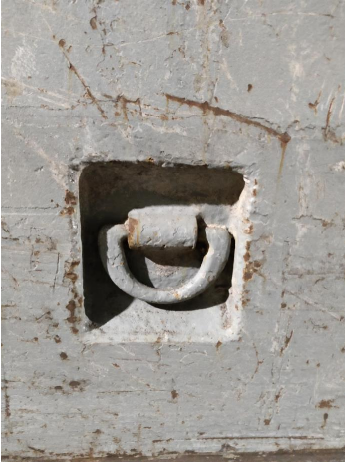
Figure 18 Side plaiting lashing point. Showing little cargo residue between plaiting and lashing ring (Matti Heinonen 2021)
