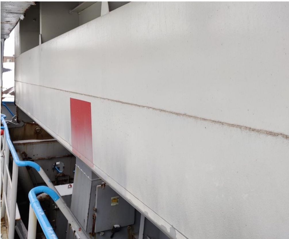
Figure 27 Intact paint on hatch cover. (Matti Heinonen 2021)
