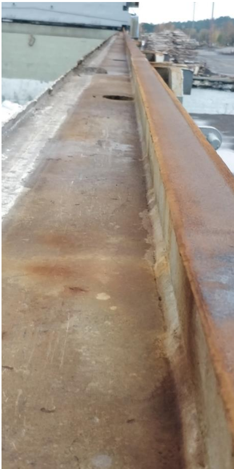
Figure 32 Hatch coaming and trackway. (Matti Heinonen 2021)
