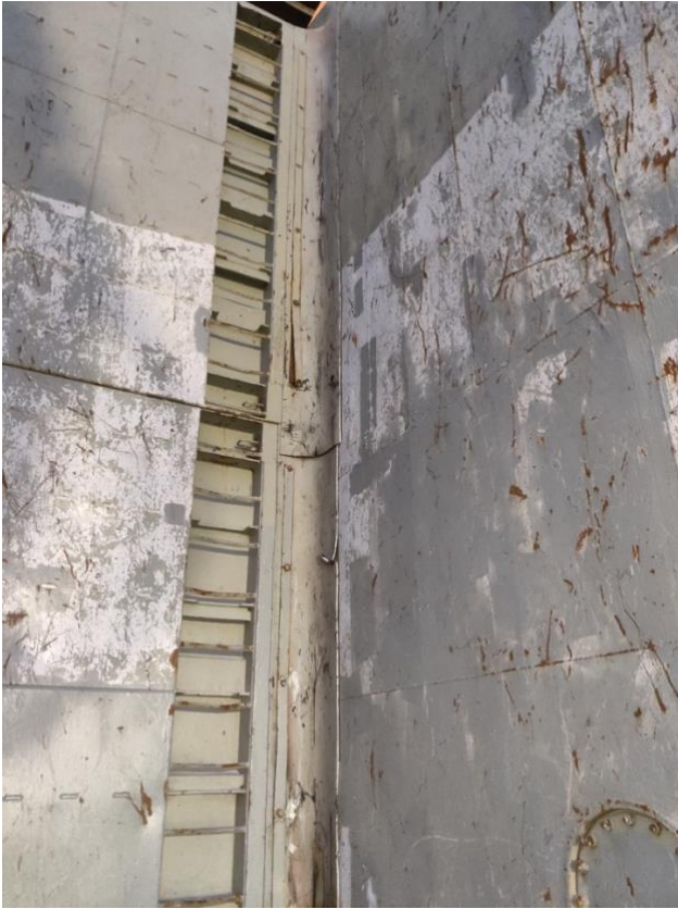
Figure 20 Bulkhead ladders (Matti Heinonen 2021)
