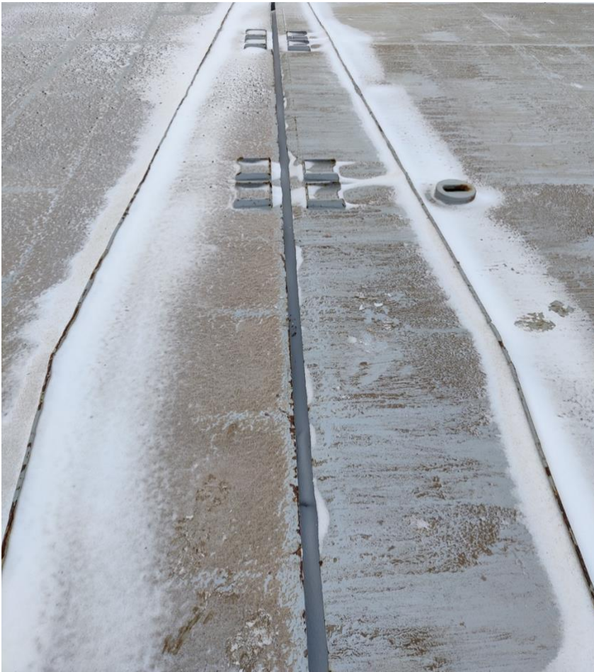
Figure 28 Snow in joint between aft and forward hatch cover. (Matti Heinonen 2021)
