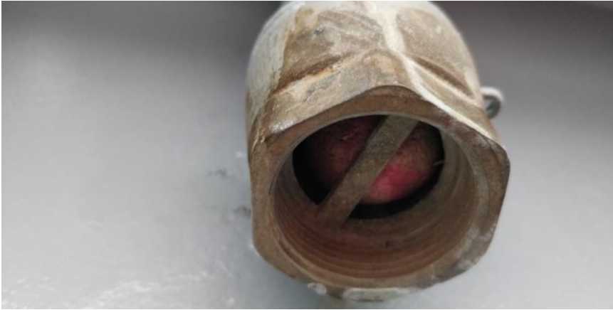
Figure 34 Draining valve. Ensure that ball inside is moving. (Matti Heinonen 2021)
