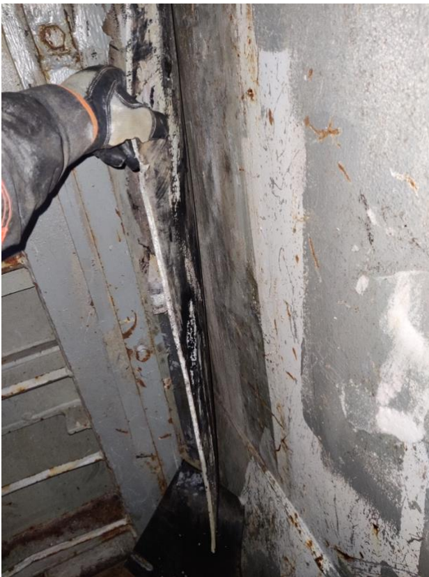
Figure 21 Check behind the rubber rug. (Matti Heinonen 2021)
