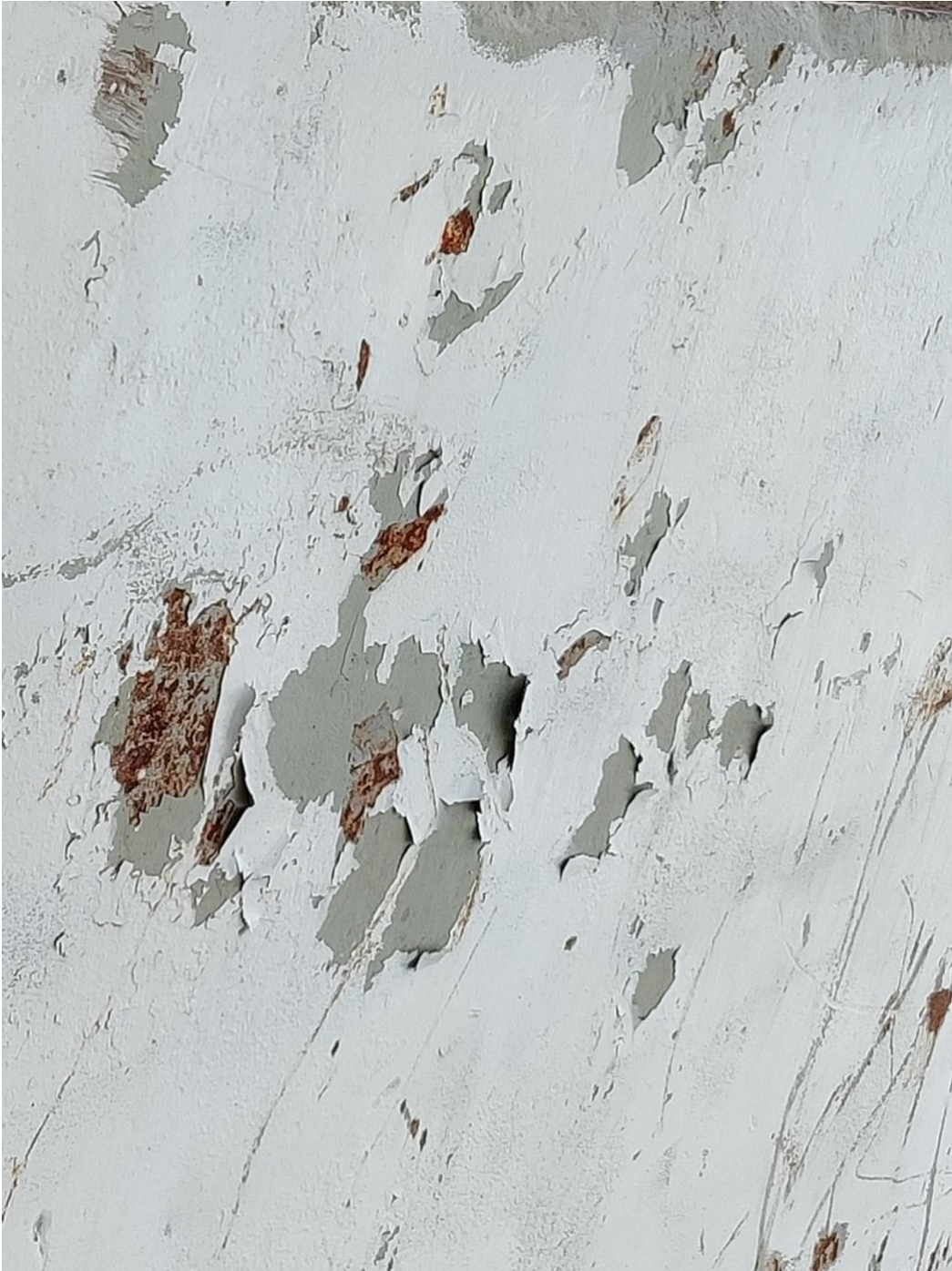
Figure 3 Loose paint side of the cargo hold (Matti Heinonen 2021)
