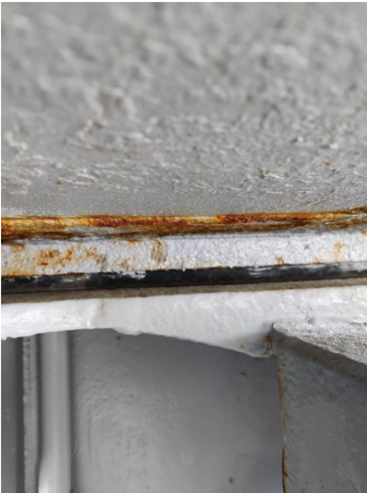
Figure 31 Closed hatch cover showing rubber packing against coaming. (Matti Heinonen 2021)
