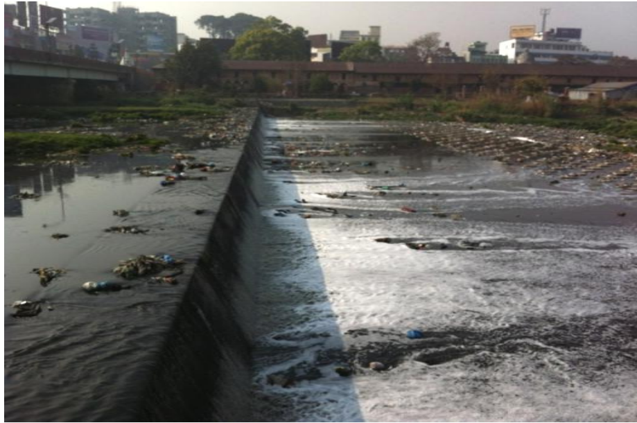
FIGURE 8. Concrete check dam under the bridge, where flow can be designed for river restoration
