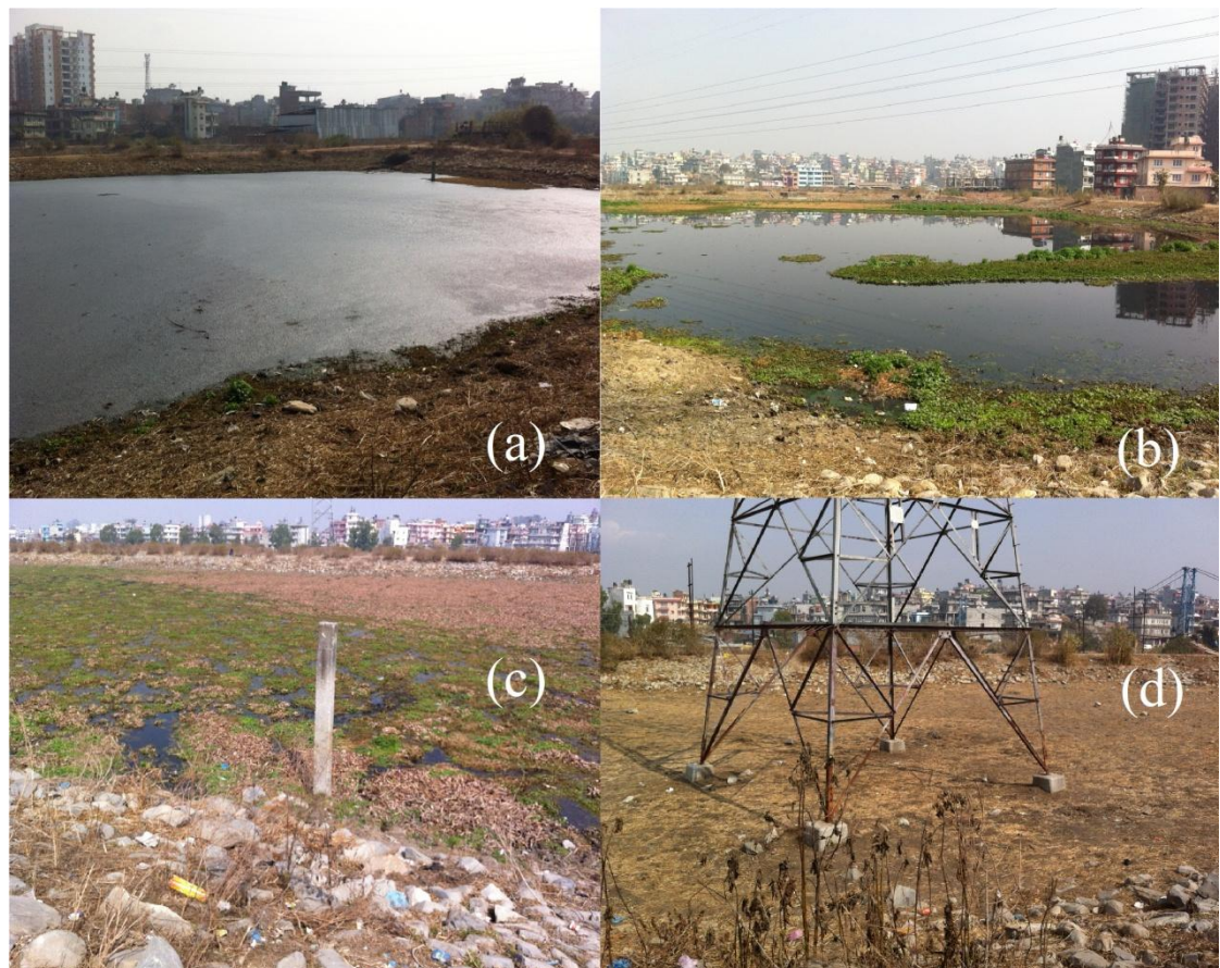
FIGURE 2. Kodku Non-aerated Lagoon WWTP; (a) First pond; (b) Second pond; (c) Third pond; and (d) Fourth pond
