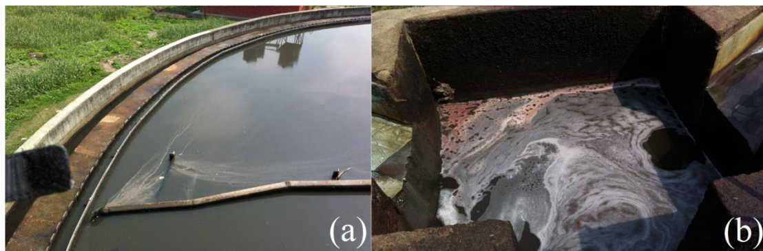
FIGURE 18. Secondary units of Guheshwori WWTP; (a) Scum removal in secondary settling tank; and (b) Foaming in effluent from Guheshwori WWTP
