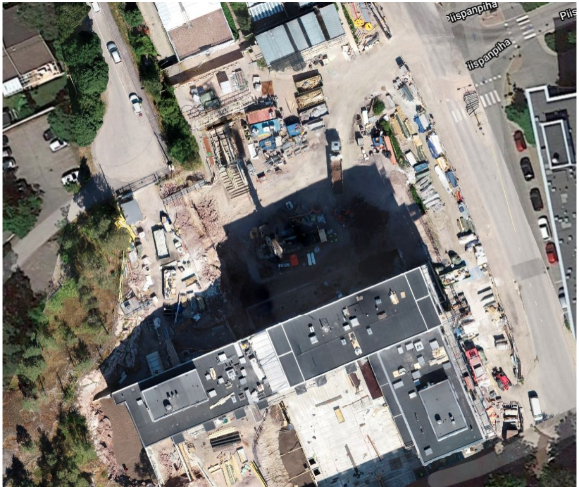
Figure 16. EKE Helmi construction site top down image.
