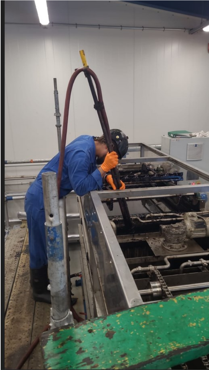
Figure 2 Laborer performing maintenance from the scaffold
